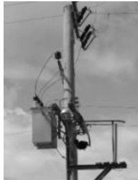
Transformers can step up or step down Voltages with high efficiency. Effective inductors require **changing** currents so A.C. electricity is used for distribution of mains electricity (except for across Cooks Strait which is no longer Level 3)
